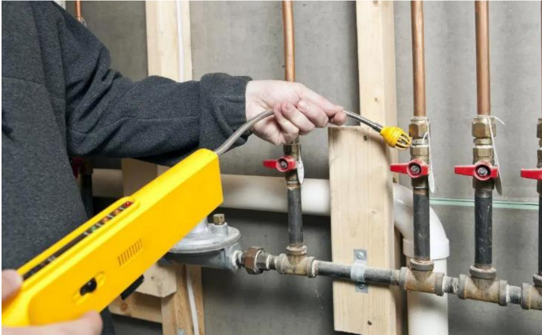
Figure 2: Gas leakage identification process [5]
